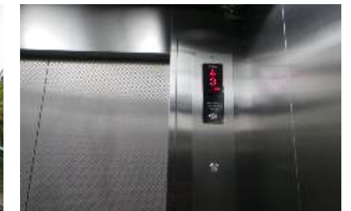
Generator back-up & Lift Facility*
