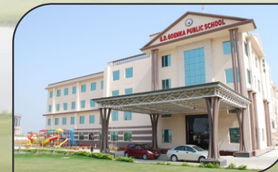
Actual picture of G.D. Goenka Public School (Operational)
